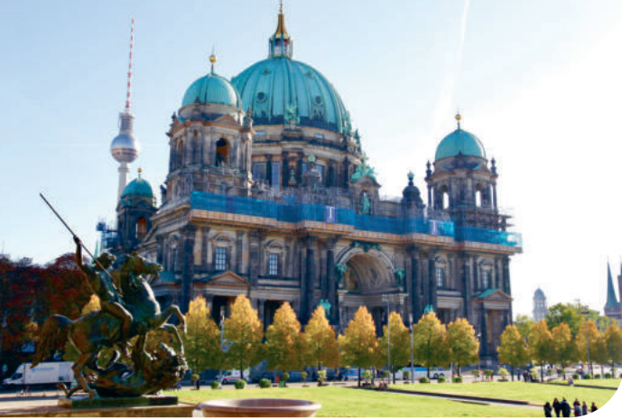
The Berlin Cathedral: Wartime damage repaired by 2008
